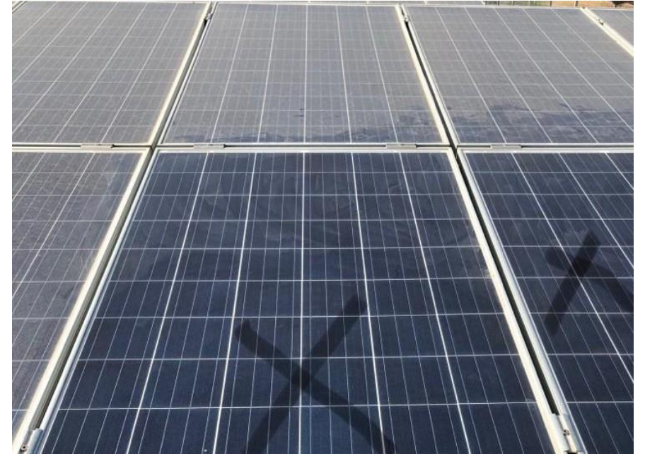
Photo one month after coating without cleaning in the Middle East
