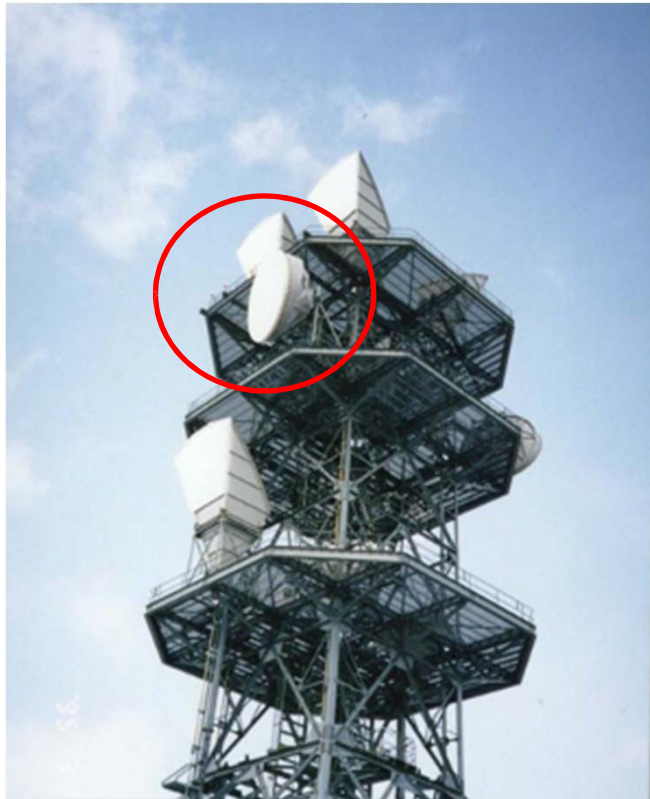
NTT radio relay tower
